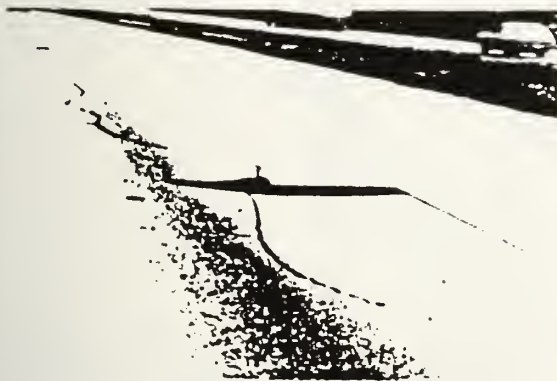
Fig. 3.2.4.2 — Meandering crack
